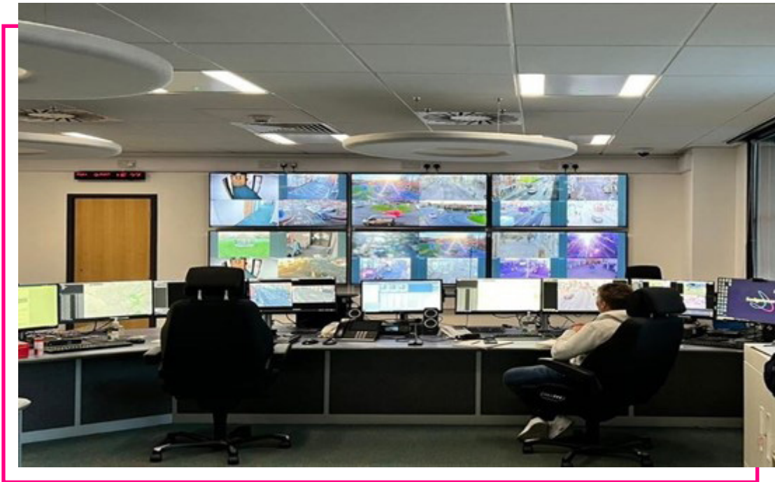
Sedgemoor District Council CCTV Monitoring Office
